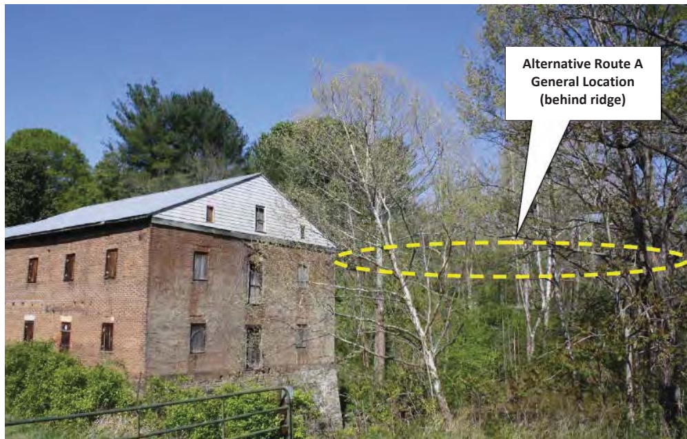
Photo 10. Galts Mill Complex Facing Northwest, Alternative Route A
