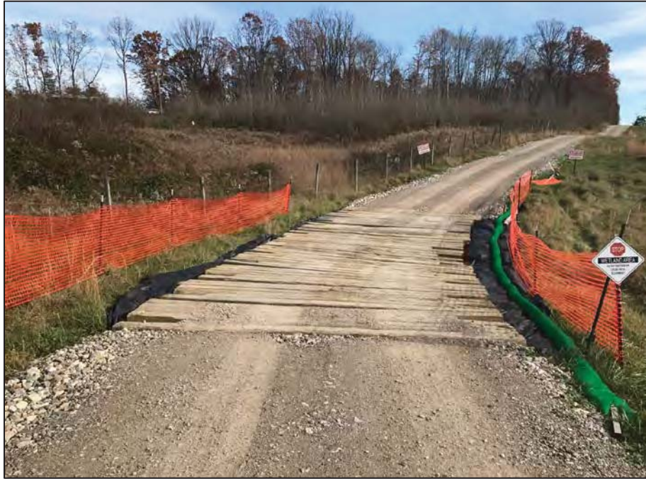
Figure 3. Typical Access Road Construction Activities
